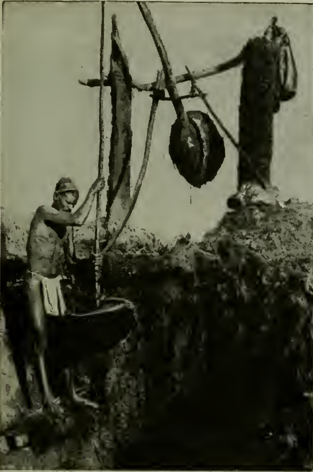
A peasant in India raising water by an arrangement known in that country as a denkli. In Egypt this contrivance is called a shadoof.
